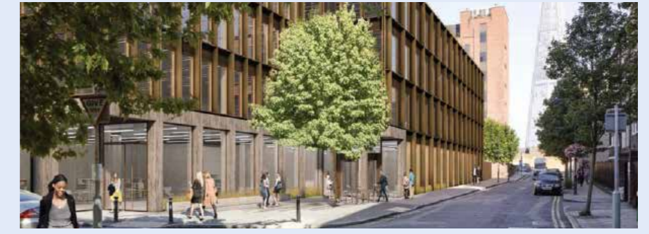
▲ The Forge, Sumner Street is the first net zero carbon P-DfMA commercial office facility in the world
